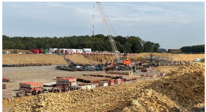
Construction of the 'Nature Bridge'
