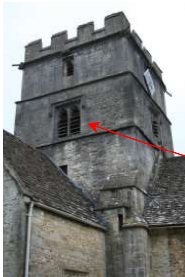
Fig 300 – South side of tower. Free stone top layer with crenellations above. Middle storey part rubble, part free stone with late perpendicular/Tudor bell openings. Lower level rubble built. Demonstrates top 1 ½ storeys rebuilt probably in late 15 th /early 16 th C. Blocked window in lower stage of tower shows south transept built later. South wall of naïve shows butting joint between 13 th C nave stonework & 12 th C tower stonework.
