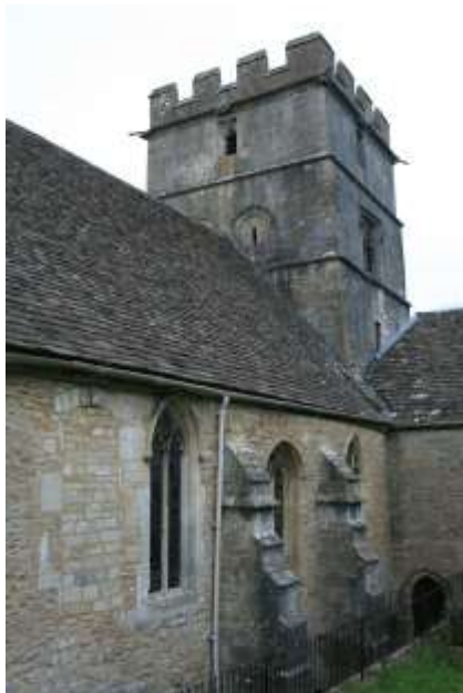
Fig 306 – west face of tower. Note 2 Norman C12 th in second stage of tower suggesting that west 2 nd storey did not need rebuilding in C15 th /16 th .
