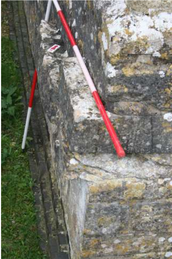
Fig 3432 – showing the kerb stones before the deepening of the trench.
