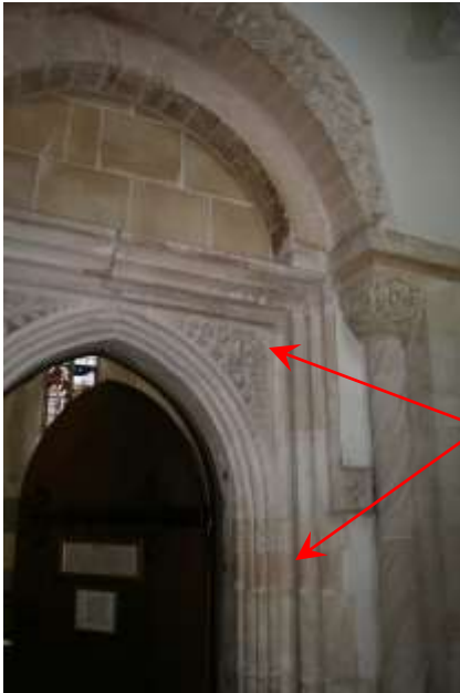
Fig 314 – North interior door; originally exterior. Romanesque columns & decorated capitals with plain round head and 15 th /16thC inset doorway.
