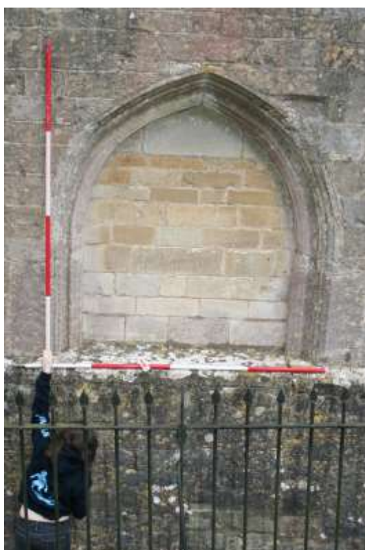
Fig 3430 – filled in door.
