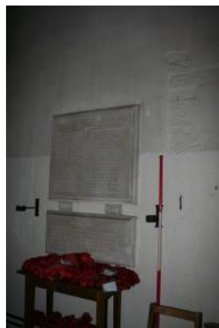
Fig 3405 – the filled in door on the west wall of the nave.
